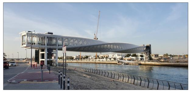
Figure 5: Steel Twisted Truss Bridge, Dubai Water Canal. (Source: Jung, 2020).
