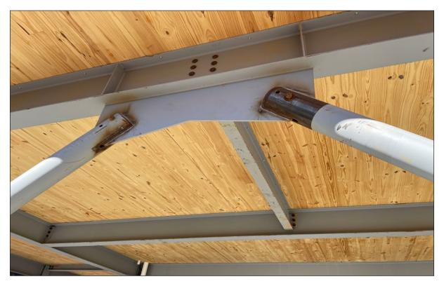
Figure 3 Wood-steel hybrid structure (Tonelli, 2022).
