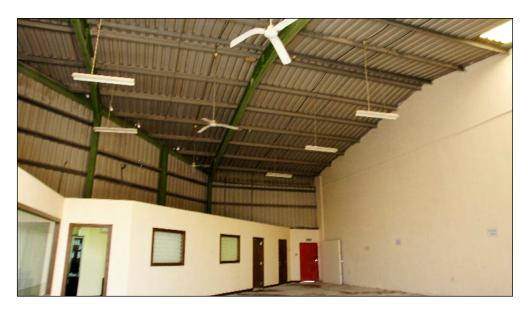
Figure 4 Mixed conditioned space. The offices at the bottom of the picture are cooled; the remainder of the interior is not (by author).
