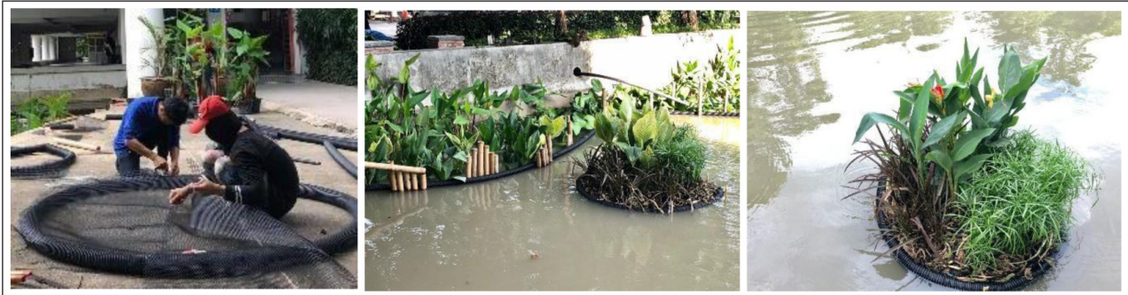
Figure 2 A design on the floating wetland beds with discarded PET plastic bottles framed with drainage pipes and geotextile.
