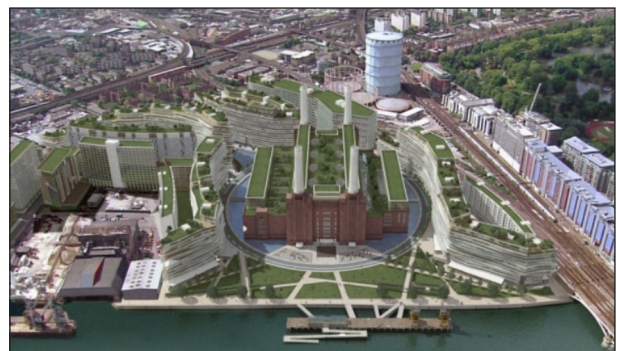
Figure 20 London recreational area near Battersea power station after its renovation.
