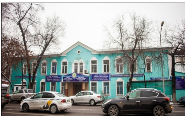
Figure 10 The building of the Almaty Financial and Legal College after renovation.
