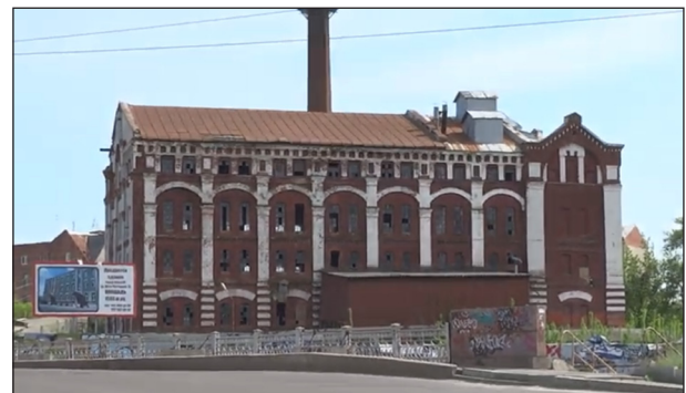
Figure 13 Unused building of the Kharkiv flour mill in Ukraine.
