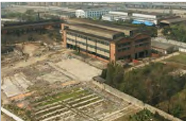
Figure 17 Large industrial building in an abandoned state.
