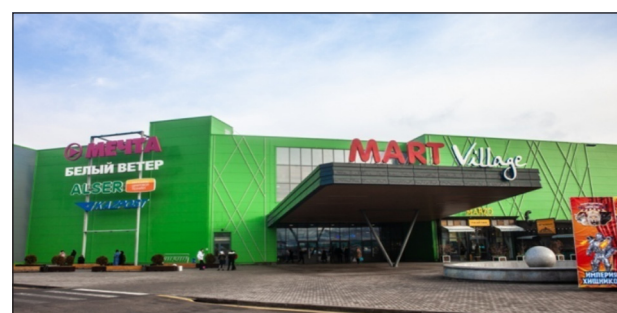
Figure 8 The AETF building after the renovation of the shopping center “Mart”.
