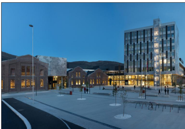
Figure 22 The Kobling Complex at the University of Bergen.
