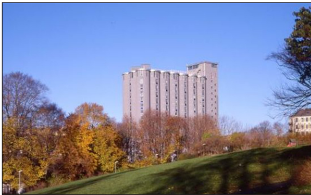
Figure 21 Grunerlokka dormitory – building of the former grain elevator.
