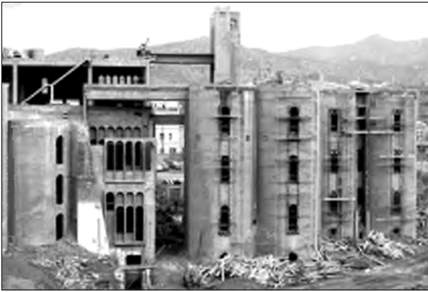
Figure 15 Factory Barcelona before renovation, Spain.
