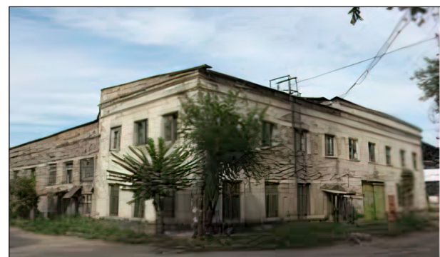
Figure 7 The AETF building before the renovation.
