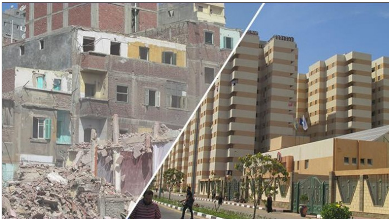
Figure 2 Ghett El Ennab before development (Left side), Bashayer El Khier 1 (Right side).
