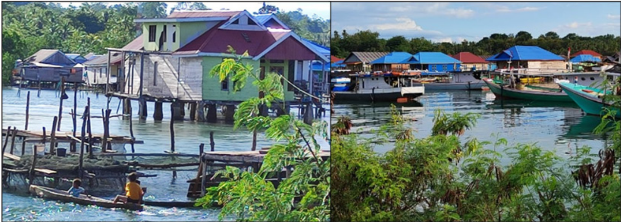
Figure 7 Various types of roof shapes on the Bajotribe houses in Lagasa village.
