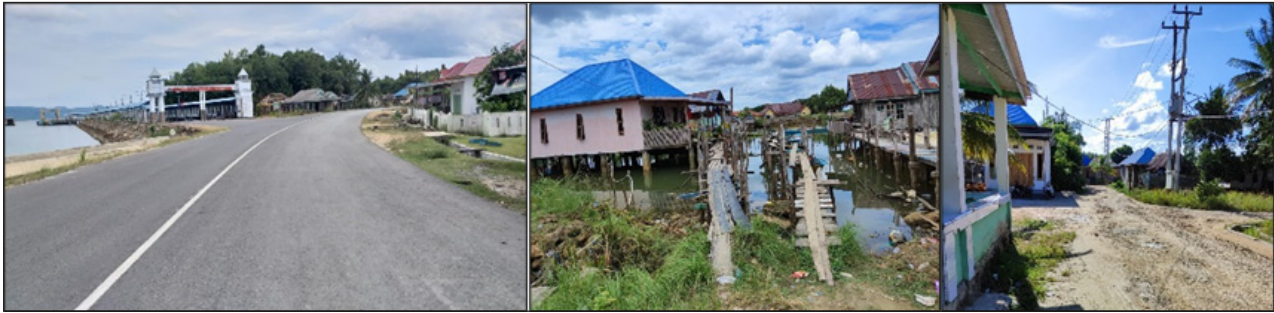
Figure 9 Conditions of main access roads and local roads in the residential area.
