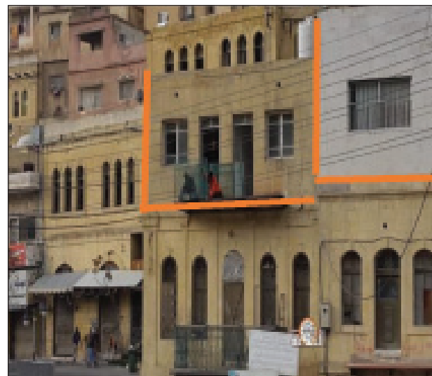
Figure 2b Extensions to original building. Source: Fieldwork.
