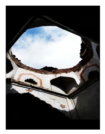
Picture 7 Heavy Rains Collapsed Masonry Dome.
