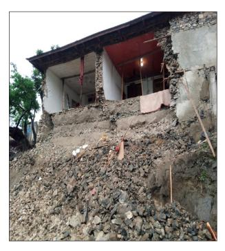
Picture 13 Damage to House in Landslide.
