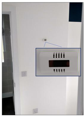
**Figure 1:** An EnOcean temperature and relative humidity sensor installed in one of the properties. A magnified view is shown in the inset image.
